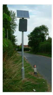
In December 2005, as part of a trial of vehicle activated signs (VAS) around the City, one of these signs was installed on Straight Lane, facing traffic approaching the village from the A166.
