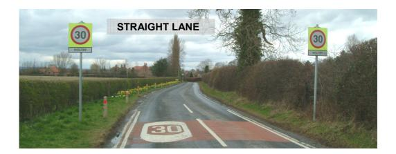
Vehicles approaching Holtby from the A166 along Straight Lane are slowed to some extent when turning off the main road before entering the 30mph limit 'gateway'. However, drivers then have relatively good forward visibility through the slight bends ahead with no roadside footway, and there appears to be little incentive for drivers to moderate their speed after entering the 30mph limit.
